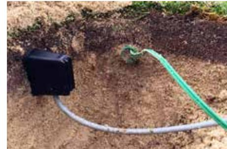
Laying the cable - inserting the sensors in the main turf root zone.
