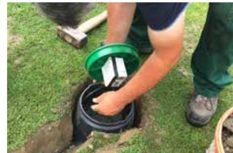
Preparation of the irrigation box for the data logger.
